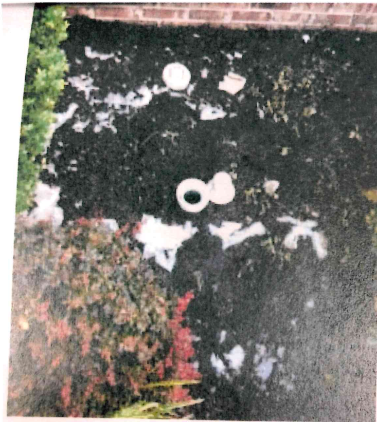
Back flow Valve Next Day - Notice Toilet Paper with Sewage
